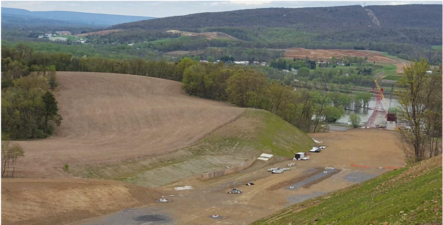
CSV T Northern Section (looking north across river and PA 147)
